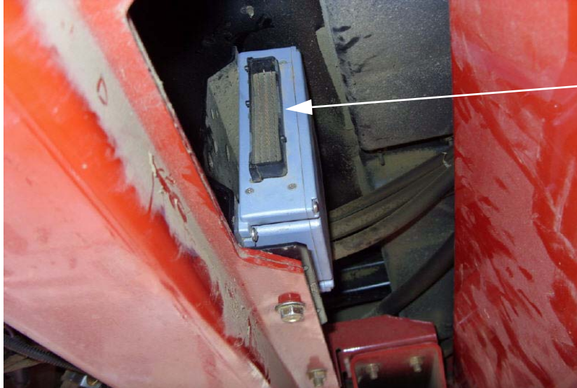
Figure 7-1 SA Module Harness Cables Bundled with Electrical Tape
